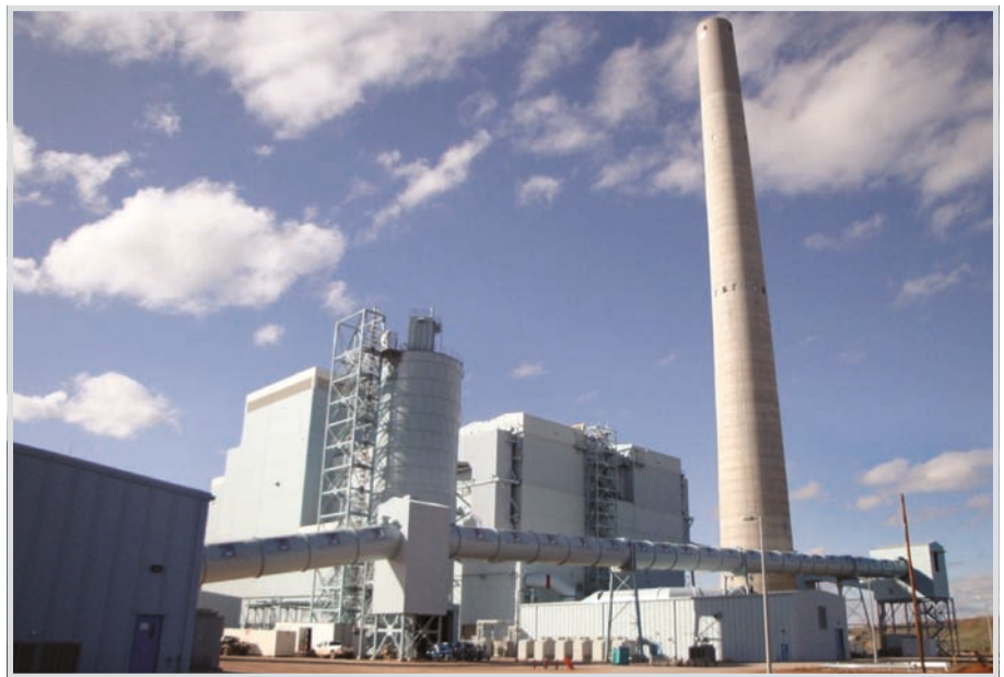
Fig. 5. World's largest CFB scrubber. The 420 MW-rated (500 MW equivalent gas flow at its 4,430 ft. site elevation) coal-fired unit at Basin Electric's Dry Fork Station has operated the world's largest CFBS since it entered service in June 2011. Since it went into operation, the CFBS has exceeded its design performance reducing SO 2 by 95. to 98 % to levels below 0.06 lb/MMBtu (50 to 60 mg/m 3 ). It also passed a 30-day mercury removal compliance test by meeting the permitted emission limit of 20 lb/TWh (2.35 µg/m 3 ) while demonstrating an Hg removal rate in excess of 95 %. Courtesy: Basin Electric Co-Op and Wyoming Municipal Power Agency.
