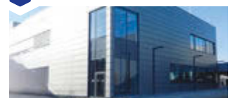
Opening of the ultra-modern Development and Technology Center in Metzingen
